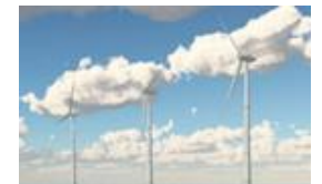
Wind Power generation
