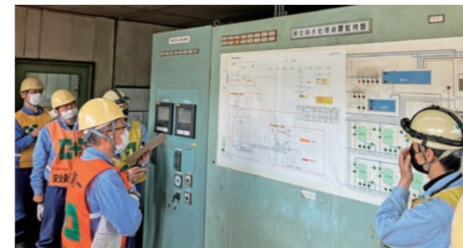
Patrol of wastewater treatment facility
