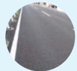
Road using electric furnace slag products
