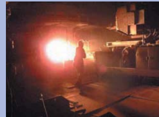
Electric furnace operation
