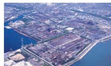
Complete View of our Head Office / Works
